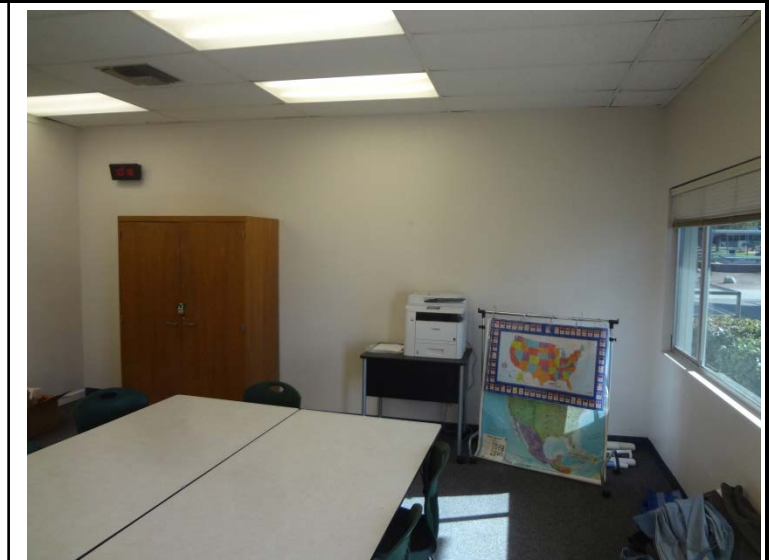
Photo -20 Underutilized Portable Classroom Portable classroom building, currently under utilized.
