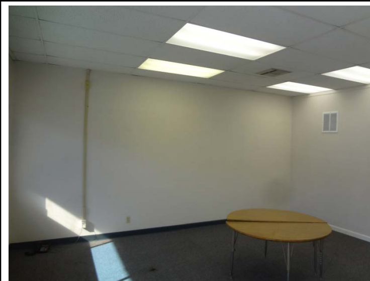
Photo -19 Underutilized Portable Classroom Portable classroom building, currently under utilized.
