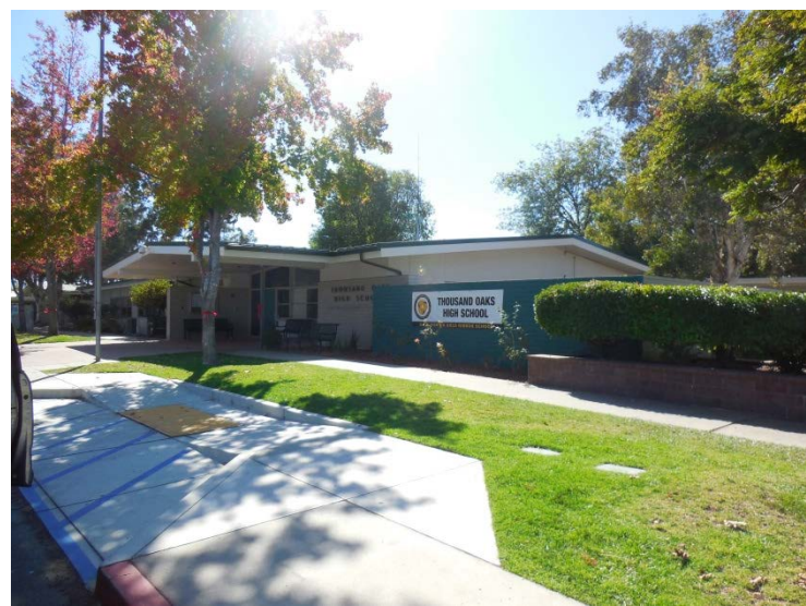
Photo -1 Curb Appeal – View of Administration Site has mature and well maintained landscaping, which highlights the administration building and marks the entry to the school
