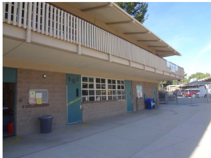
Photo -5 Curb Appeal – View of Classrooms Classroom buildings have split face CMU finish and large balconies that wrap the second floor.
