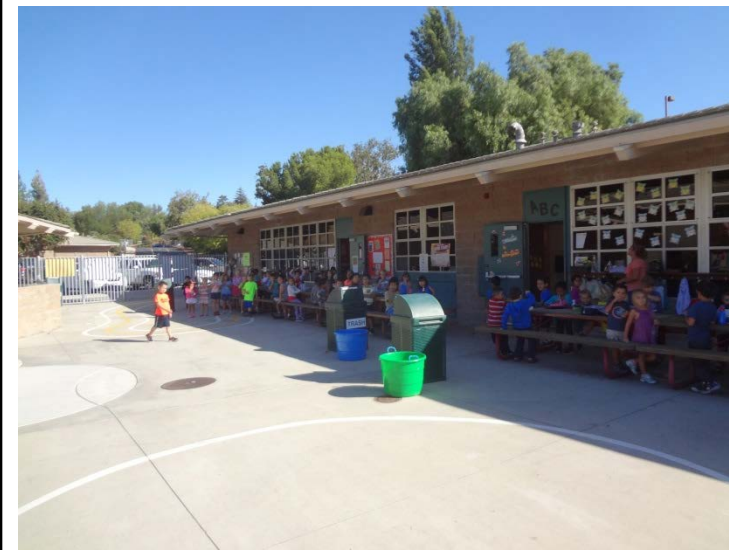
Photo -3 Curb Appeal – Kindergarten Kindergarten classrooms have split face CMU finish with large overhangs that shade picnic tables for the students to enjoy the outdoor environment.
