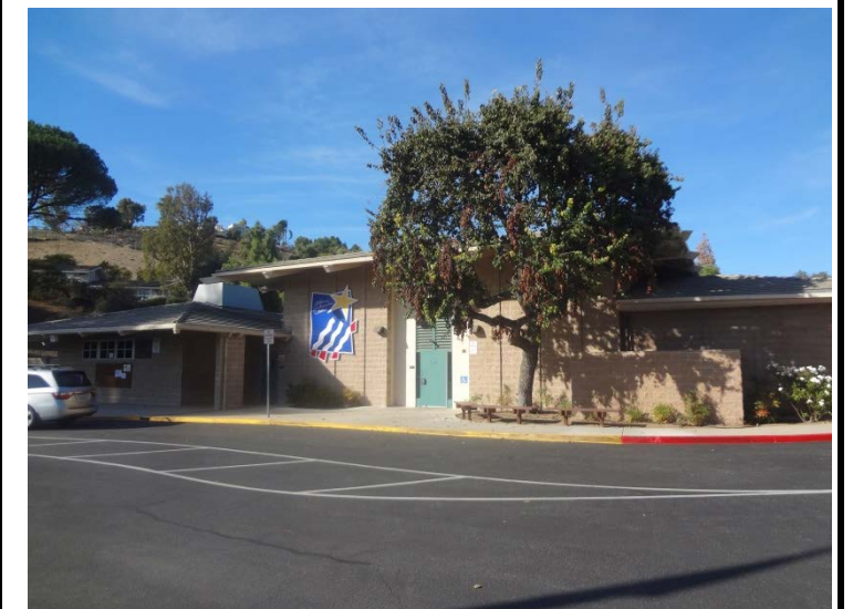
Photo -8 Curb Appeal – View of MPR Large MPR has split face CMU finish with mature trees and foliage.
