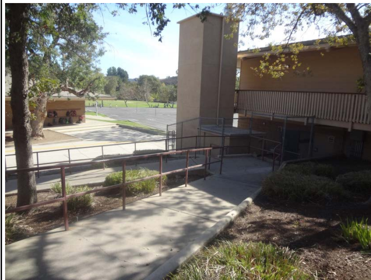
Photo -2 Curb Appeal – View of Ramp Ramps on campus are well landscaped, shaded and frame different views in the distance with tree canopies.
