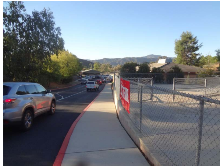
Photo -2 School Parking Entry Long Steep sidewalk to school entrance poses a challenge to people in wheelchairs.
