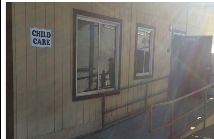
Photo 7 Building Name: Portable Classroom Building Number: 5 Description: 40x40 Child Care Center
