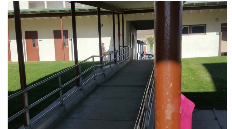
Photo -4 Ramp does not appear to comply with current accessibility standards.
