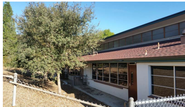
Photo 14 Building Name: Classroom Building Number: 12 Classroom building at the bottom of a steep grass hill, which poses drainage concerns during heavy rains.
