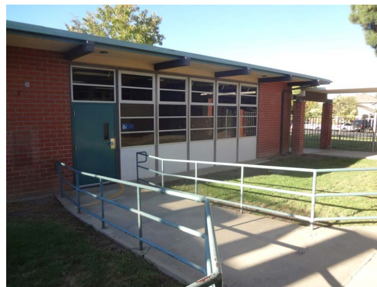
Photo -6 Building 8 Backside of learning center building with possible transite panels, and windows between primary brick structural systems and a sloping ramp between building 8 and 7
