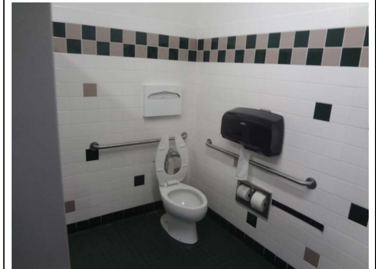
Photo -24 Building 4 Typical public restrooms for students have received accessibility upgrades
