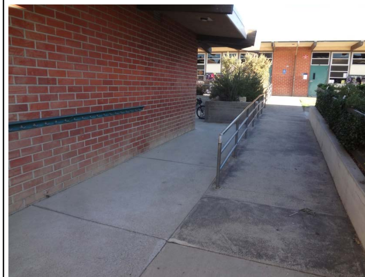
Photo -7 Building 1 Accessible ramp from Building 1 to Building 4
