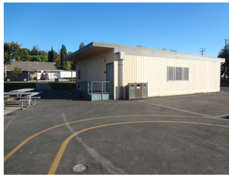
Photo -2 Building 6 Typical modular classroom building with wood panel façade finish.
