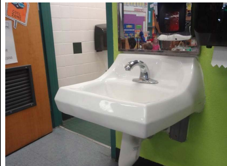
Photo -15 Building 7 Accessible sink in kindergarten classrooms
