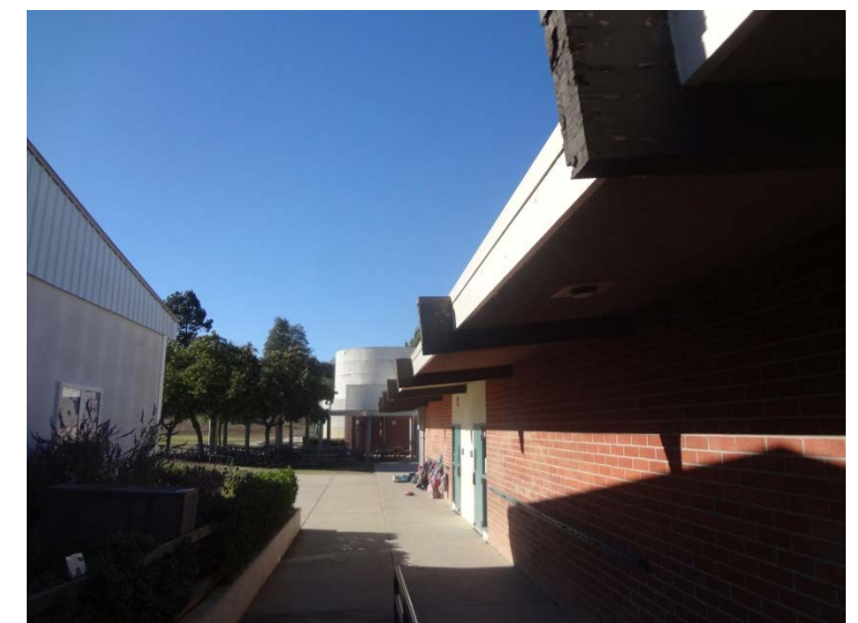
Photo -8 Building 1 Backside of building 1 looking toward multi purpose building
