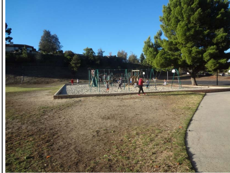
Photo -19 Playground Area Playground equipment is not shaded, but otherwise in decent condition. There is no accessible path to equipment.
