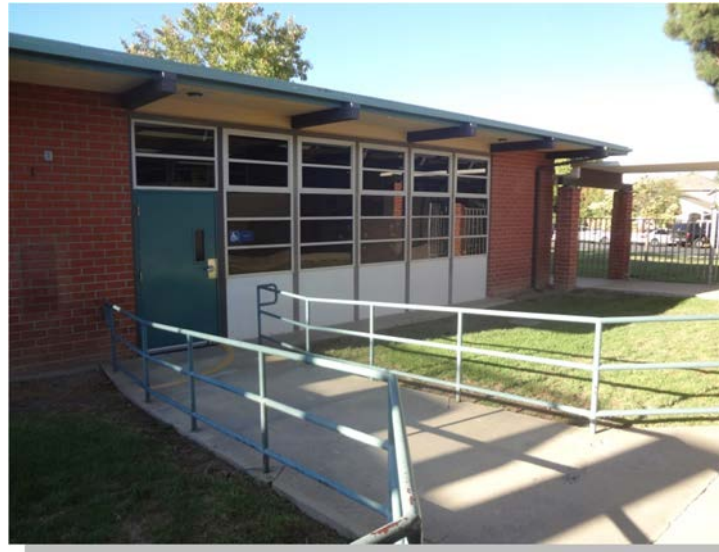
Photo -1 The ramp leading to the learning center is current with accessibility standards. It does not have the proper landing size
