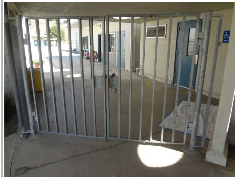
Photo -3 Gates to Campus Gates to campus do not have accessible hardware.
