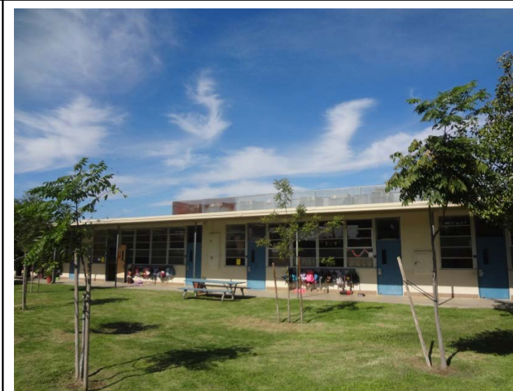
Photo -3 Curb Appeal – Classroom Buildings The classroom buildings have large overhangs that cover the walkways and shade the classroom windows
