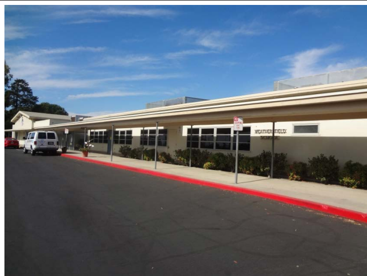
Photo -1 Curb Appeal – Administration Building Large Overhangs shade the walkways and building façades.
