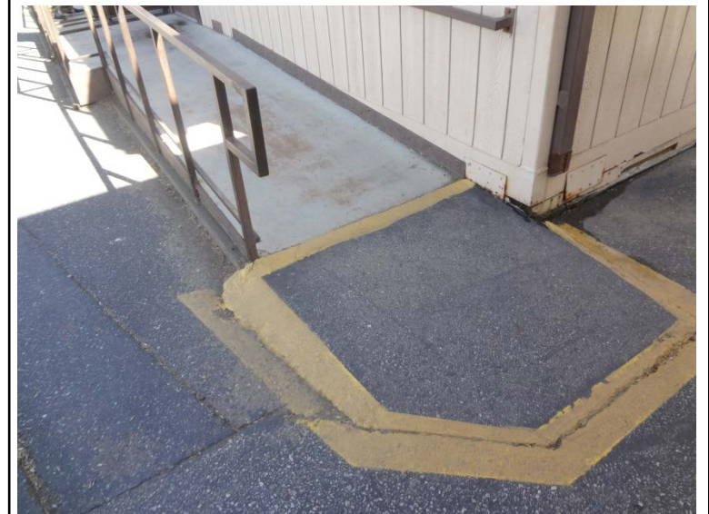
Photo -4 Portable Ramps Portable building ramps do not have compliant landings
