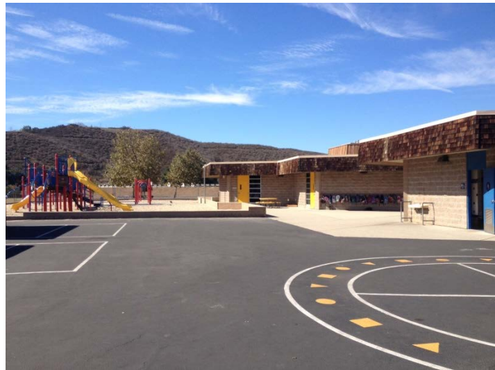
Photo 17 Building Name: Classroom Building Number: 5 View of a classroom building, with a play yard in the foreground and a portion of restroom building visible.
