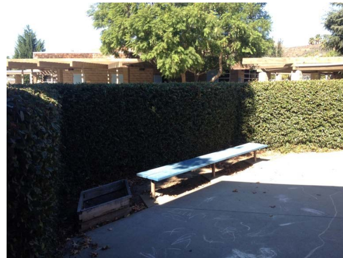
Photo 19 Building Name: Classroom Building Number: 3 Classroom building #3 has a hedge wall as a breakout exterior space.
