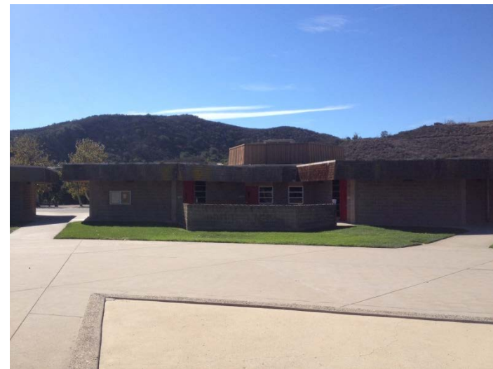
Photo 14 Building Name: Classroom Building Number: 5 Typical classroom building shown.
