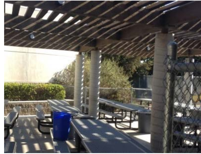
Photo 10 Building Name: Lunch shelter Building Number: N/A Lunch shelter area, facing Multi-Purpose building.
