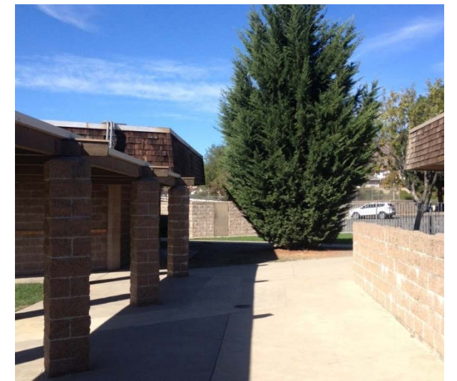
Photo 12 Building Name: Classroom Building Number: 9 Walkway between administrative building and a classroom building.
