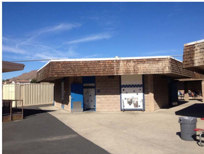
Photo 13 Building Name: Restroom building Building Number: 8 Hexagonal restroom building.
