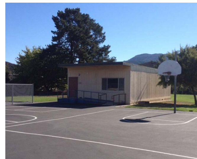
Photo 15 Building Name: Storage Building Number: 11 Previously a portable classroom.
