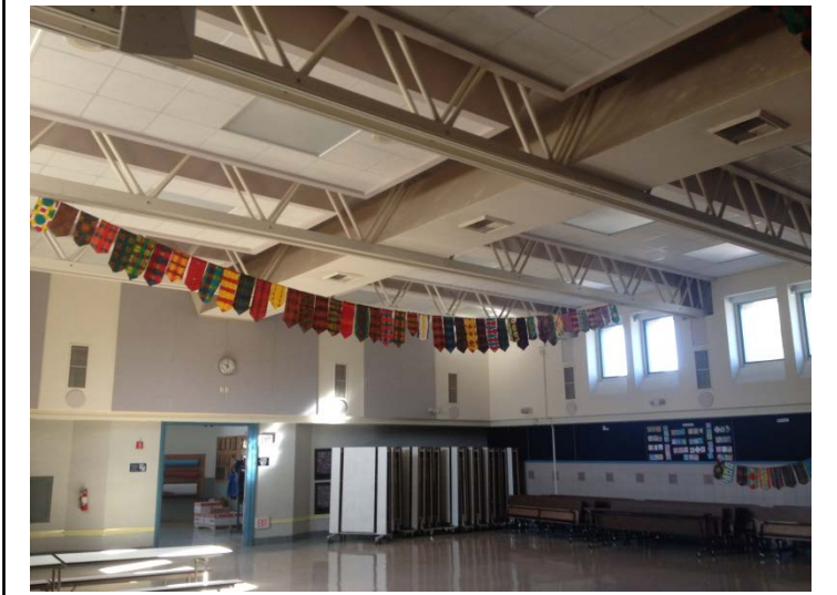
Photo 16 Building Name: Multi-Purpose building. Building Number: 2 Assembly space within Multi-Purpose building.
