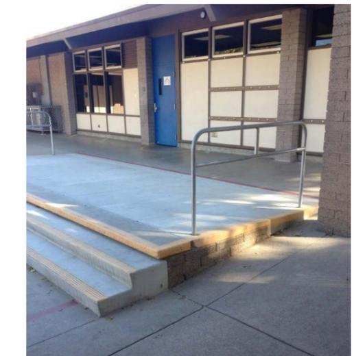
Photo 4- "Stage" in main courtyard lacks compliant stairs and handrails.
